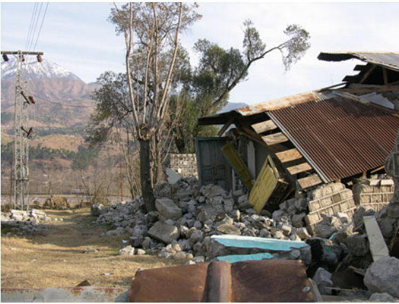
Fig. 5.2 A hospital completely demolished by the October 2005 earthquake in Muzaffarabad
